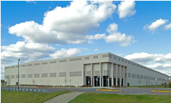
South River Road, South Brunswick, NJ
