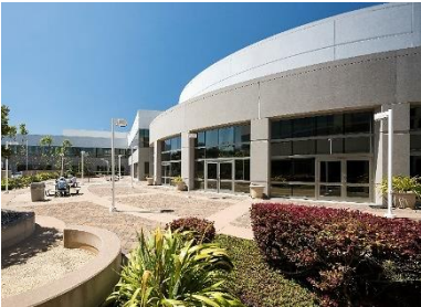
500 Forbes Blvd, South San Francisco, CA
